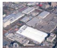
NSK Fujisawa Plant
