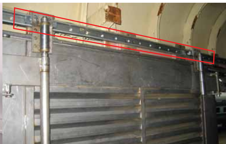
HEAVY DUTY RAIL RB 43 USED IN RAILWAY SLIDING DOOR
